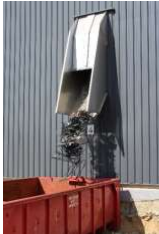
The Vidatris goes through and allows to empty the waste in the container without leaving the building
