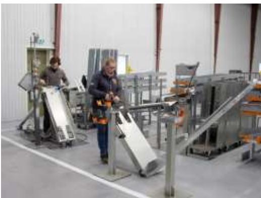
Labadis technical floor includes all cable types : ground is free and view is cleared
