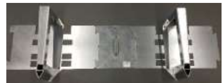
Laying template to position the sheets on the floor in 600 mm wide lines
