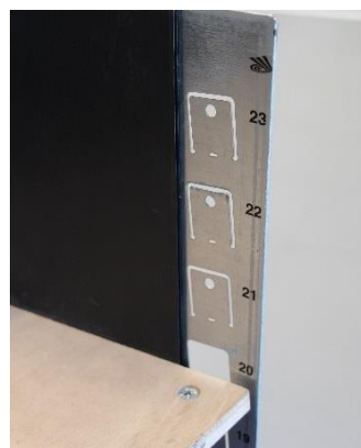
Numbered graduation guides the position of the shelves
